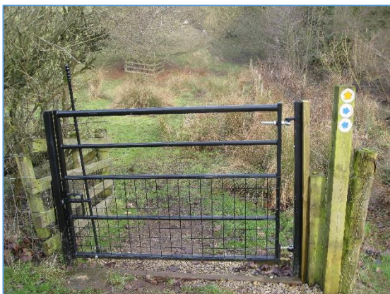
Here the bridleway is in front of the gate; only the footpath goes beyond it. Therefore, the blue waymarks are misleading and unnecessary. They should be on the other side of the gate for those approaching the bridleway from the footpath.
